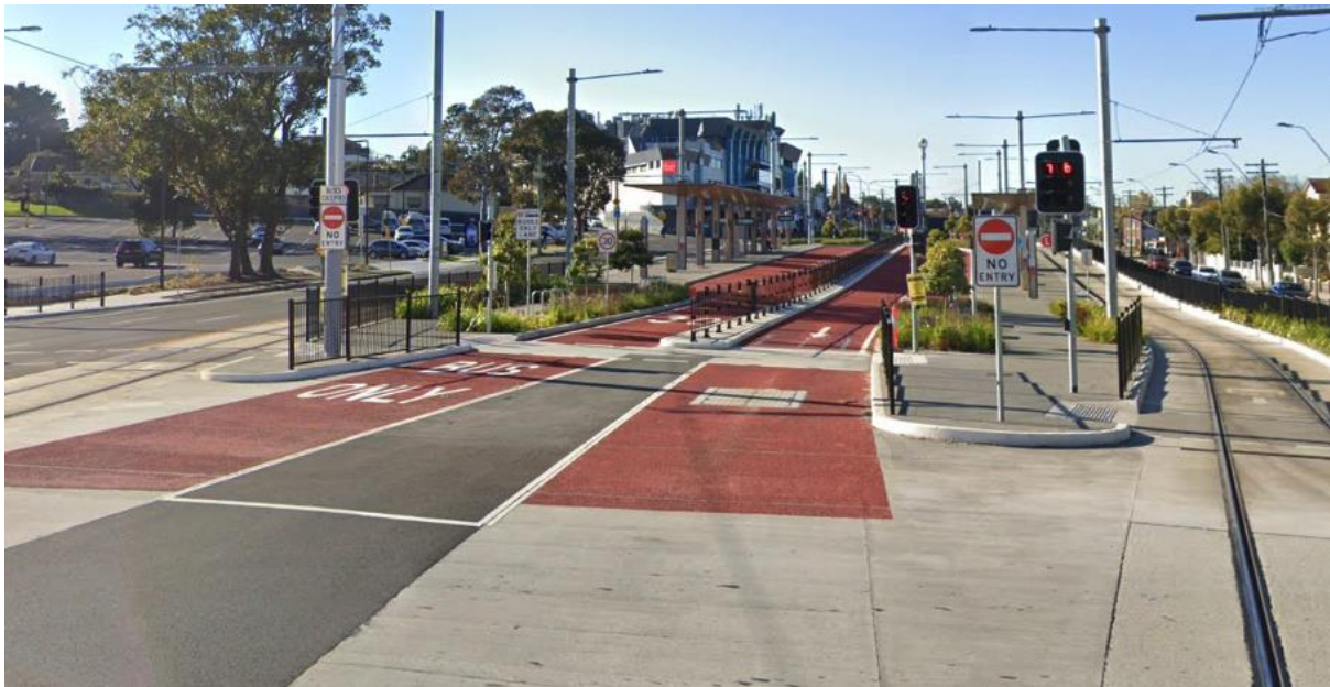
Figure 10: Souths Juniors Club at Kingsford building viewed from Anzac Parade, Gardeners Road intersection (Source: Google Maps).
