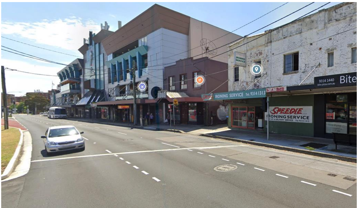
Figure 8: Anzac Parade frontage of Souths Juniors Club at Kingsford building and adjacent development looking west (Source: Google Maps)
