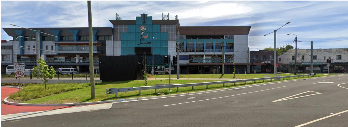
Figure 9: Souths Juniors Club at Kingsford building viewed from Anzac Parade looking north (Source: Google Maps).
