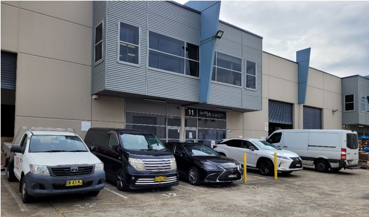
Figure 3: Light industrial complex, 133-137 Beauchamp Road, Matraville
