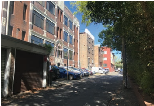
Arthur Lane - existing view looking south from Waratah Avenue
