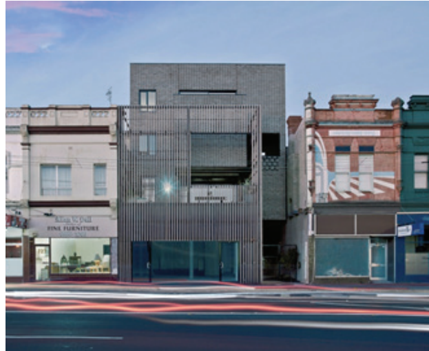
New infill with a heritage context (729 Burwood Rd, Hawthorn East, Melbourne)
