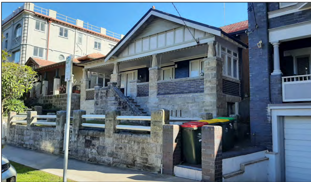
Figure 32: View of 148 and 150 Brook Street (Source: Randwick City Council)
