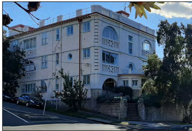
Figure 35: View of 152 Brook Street (Source: Randwick City Council)
