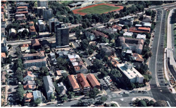
3D Image 3: View of the entire HIA from the east
