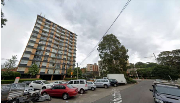
Photo 7: Abbotford Street looking southwest (Jul 2019)
