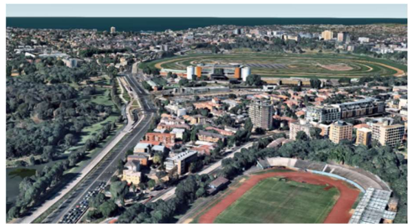
3D Image 2: Southeast view of the HIA displaying views towards Randwick Racecourse and Coogee.
