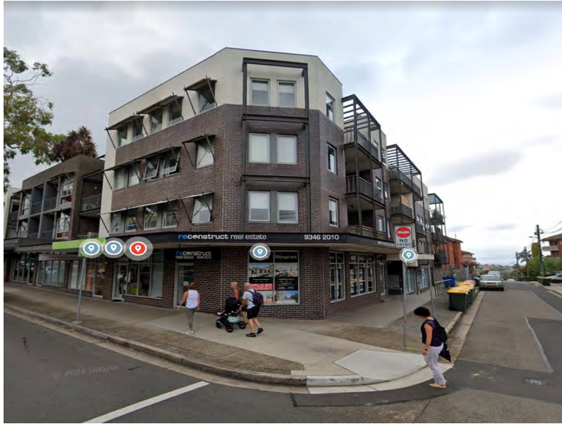
Figure 39: 155-161 Avoca Street, Randwick – an example of recent development
