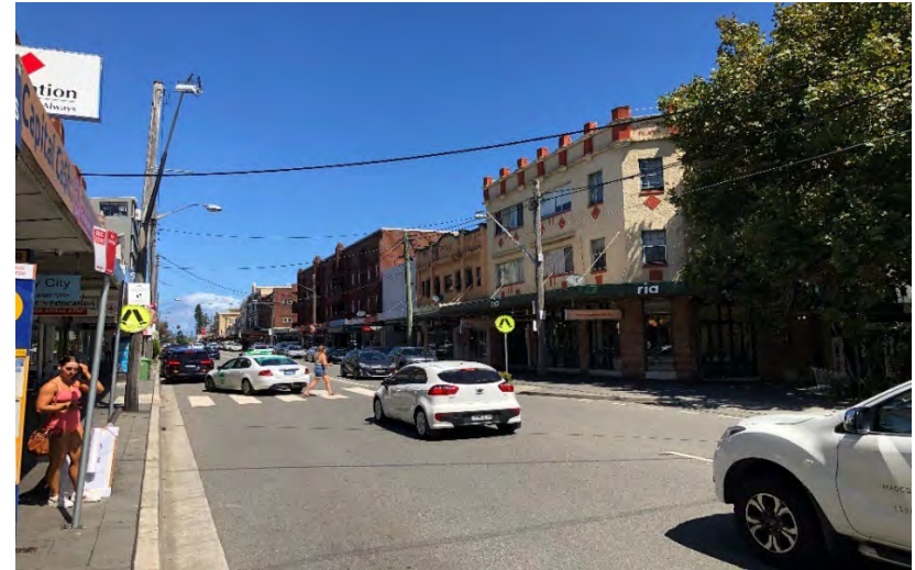
Figure 66: Current built form – Belmore Road angled view
