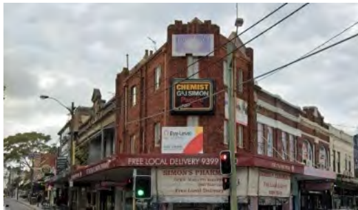
Figure 30: Inappropriate signage mounting and location
