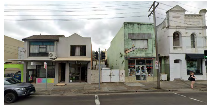
Figure 31: Dilapidated shopfronts and heritage facades on Avoca Street
