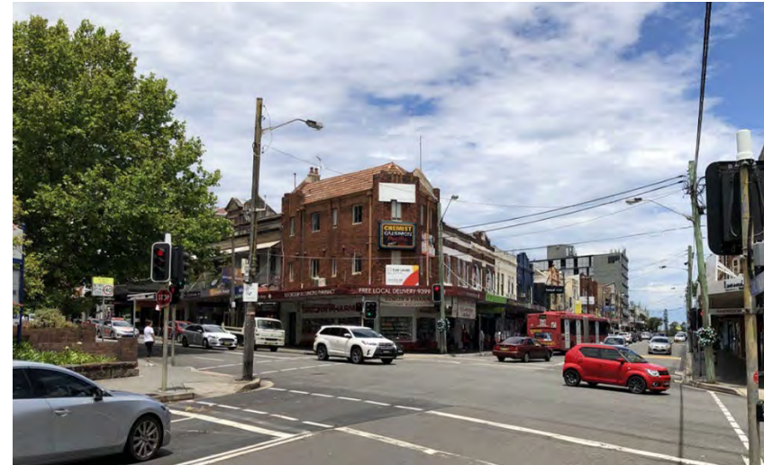
Figure 57: Existing corner of Belmore Road and Alison Road, looking south-east
